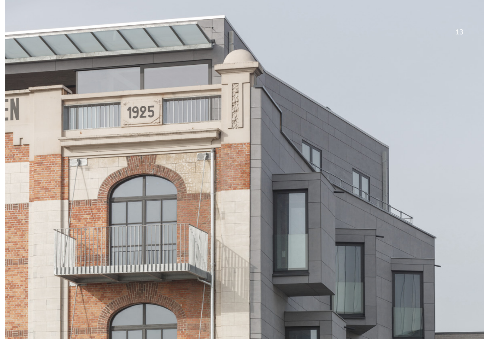
Peynsaert Architecten Aalst, Belgium | EQUITONE [tectiva]®
