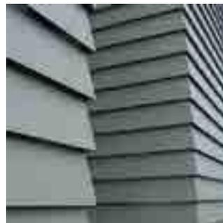
While the vertical joints are spaced at 10mm the horizontal joints overlap. These can be overlapped close to each other or special spacers are available from support frame suppliers that result in a stand-off overlap which gives a deeper shadow.
