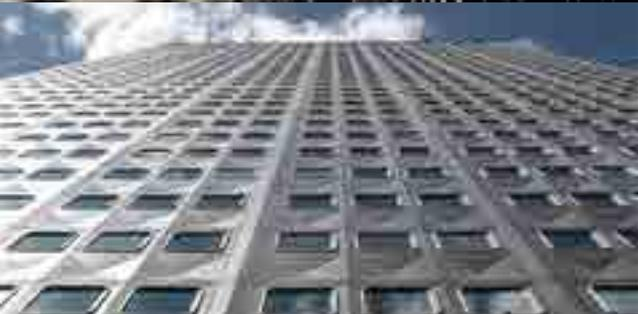
The Alcoa building in Pittsburgh, originally designed by the Architect, Harrison + Abramovitz was one of the first very large buildings to utilise modern rainscreen cladding. The 30-storey building was built in 1952 and clad with large baffled aluminium panels. The baffling provided resistance to water penetration. Ventilation was provided in the airspace between the cladding and the main wall to dry any moisture.
