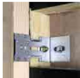
The adjustable brackets are alternately placed to the left and the right of the vertical batten. This helps to prevent the batten twisting and keeps a straight supporting frame.
