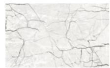
FCS 547 Cracked marble
