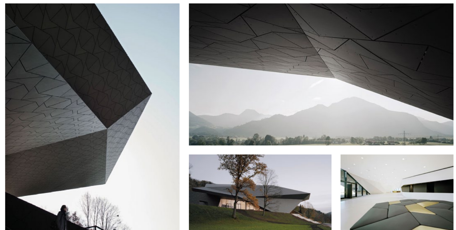
Arch.: Delugan & Meissl Architects, Austria
