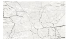
FCS 547 Cracked marble
