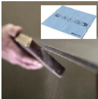
After sanding the edges of the panel remove all dust from the edges.
