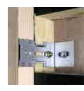
The adjustable brackets are alternately placed to the left and the right of the vertical batten. This helps to prevent the batten twisting and keeps a straight supporting frame.
